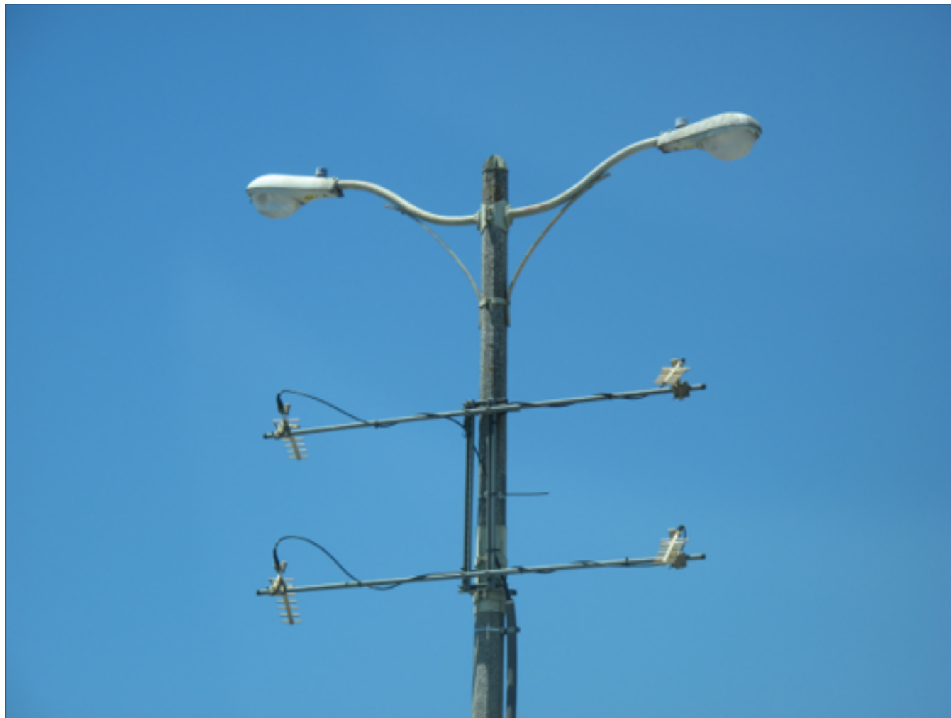
Yagi antennas pointed into each lane. This is not a toll point! This is traffic 'monitoring'.
